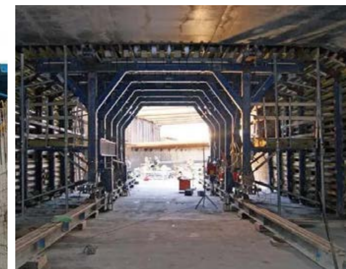
Timber Formwork Pipe Gallery Tunnel Trolley 木模体系台车
