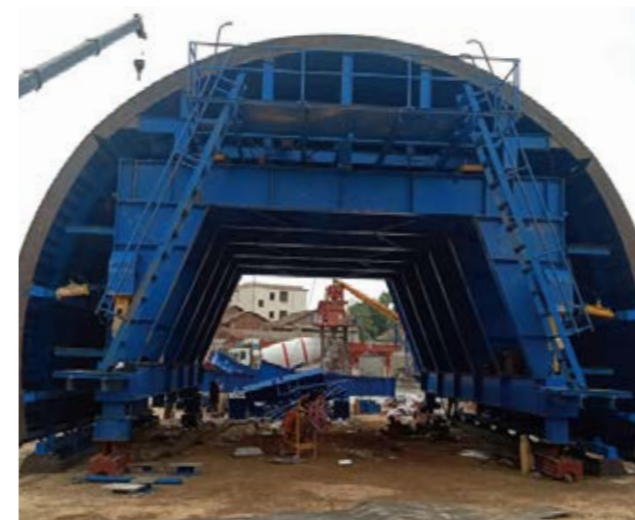
Steel Formwork Tunnel Trolley 钢模体系隧道台车
