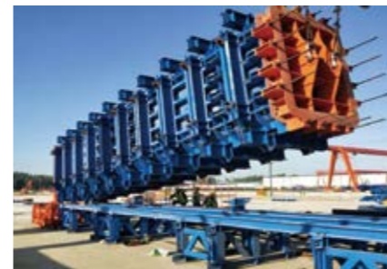
Prefabricated Pier 预制墩柱
