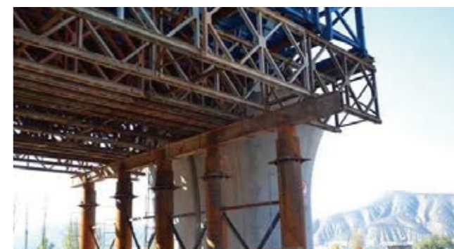
Beret Beam Support 贝雷梁支架
