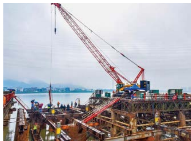
Steel Box Cofferdam with Bottom 有底钢套箱
