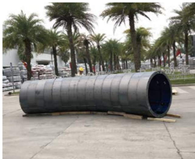
Steel Formwork for Circle Tunnel 圆形隧道钢模板
