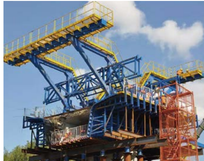
Balanced Cantilever Carriage 挂篮
