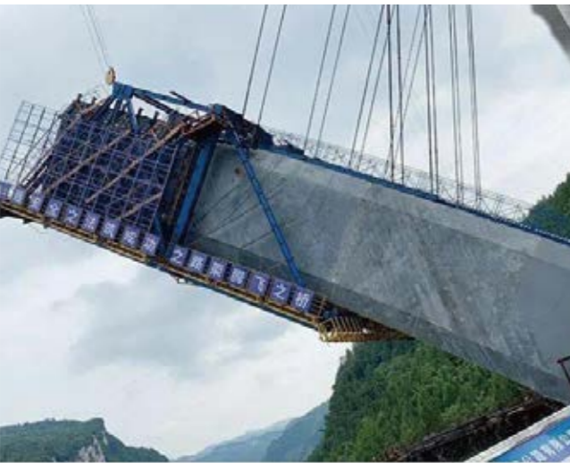
Cantilever Carriage for Arch Bridge 拱桥挂篮
