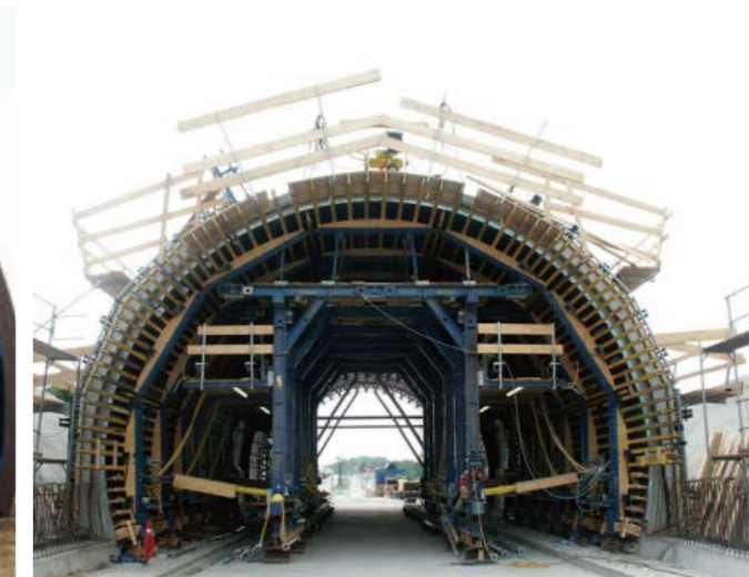
Timber Formwork Tunnel Trolley 木模体系隧道台车
