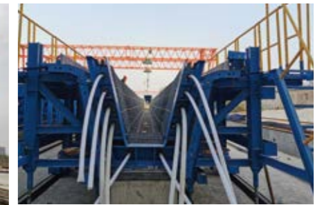
Prefabricated Box Girder (Hydraulic) 预制箱梁(液压)
