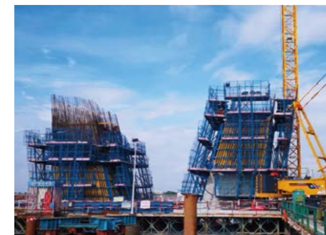
Climbing Formwork for Pier 墩柱爬模
