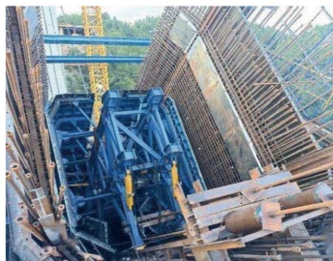
Cantilever Carriage for Arch Bridge 拱桥挂篮
